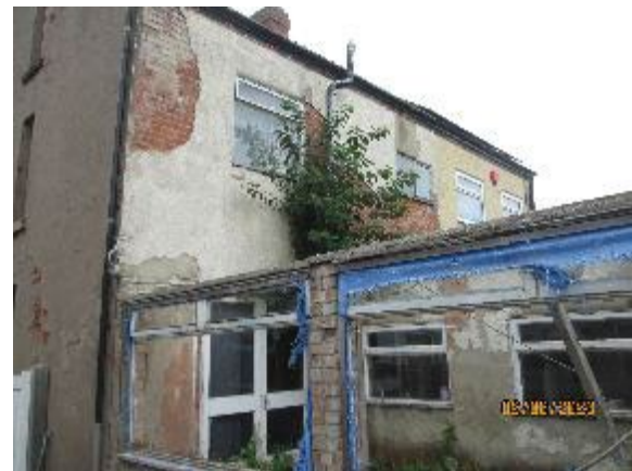
Rear elevation – some elements to be demolished
